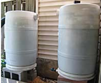
Align rain barrels on top of supports
