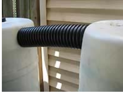
Install overflow connection tube
