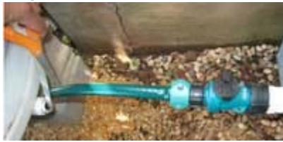
Measure, cut, install female fitting on end of garden hose
